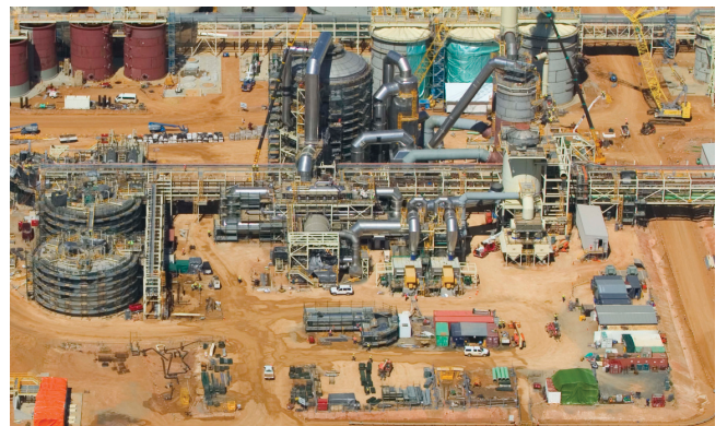
4,500 MTPD plant under construction
